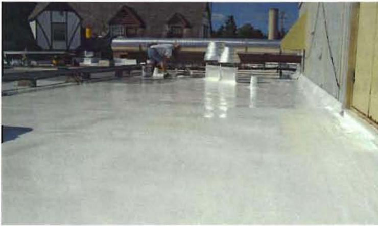
Above: Completed roof.
